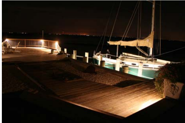
Wrightliters with yoke mount installed below bulkhead to accent sailboat and wooden dock. In the background, Postliters are mounted on deck railing on waterfront. Residence in High Bar Harbor - Long Beach Island, New Jersey Photo courtesy of Tanek Hood, Reynolds Landscaping
